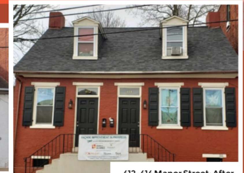
412-414 Manor Street: After
