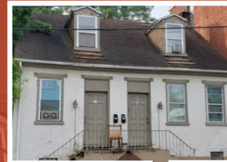
412-414 Manor Street: Before
