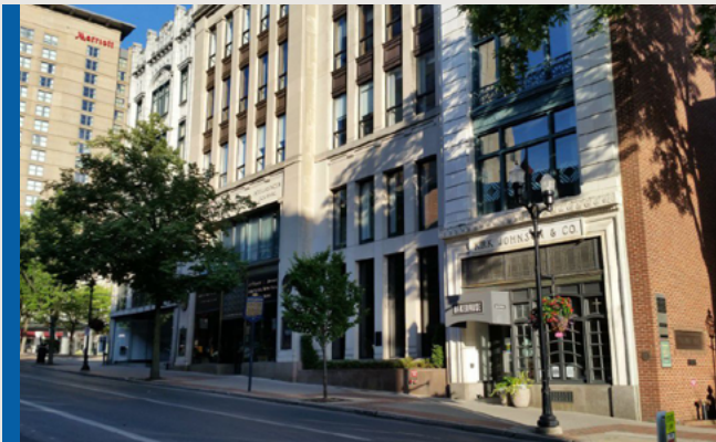
▲ The Intel (Mixed-Use) | 4–18 West King Street Under construction; anticipated completion in 2023
